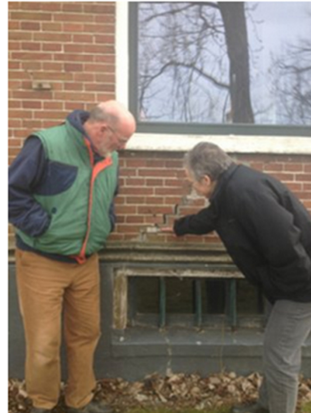
Klaas Koster and Jannette Schoorl show a crack in the wall of their home in Middelstum
